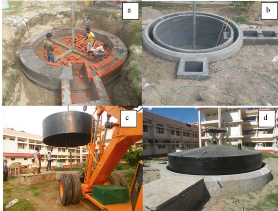
Fig 7 Different stages of the construction of the biogas plant
