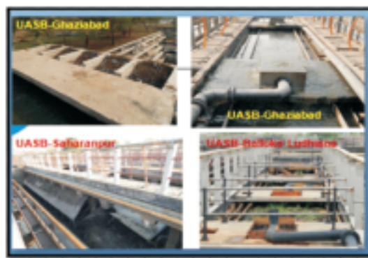
Figure 4: UASB reactors at different STPs
