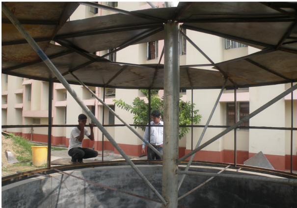
Installation of Biomethanation Plant_ A learning paleform
