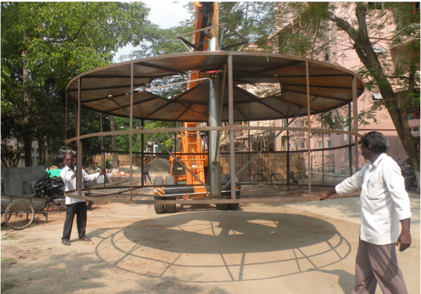
Installation of Biomethanation Plant_ A learning paleform
